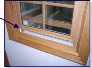
Then, raise the bottom sash approximately 3" from the sill so that the lift rail clears the dam wall while tilting.
