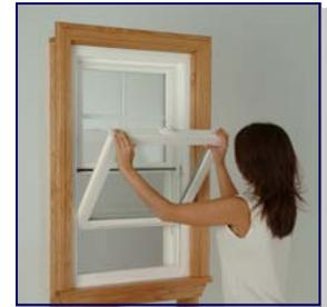
**STEP 3:** To tilt the top sash, lower the top sash to just above the bottom lift rail.
