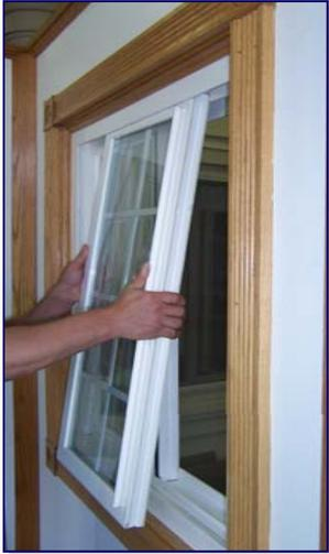
To remove the sash of Seaway's Accolade slider window for cleaning purposes, first unlock the window and slide the sash to the **center** of the window.
